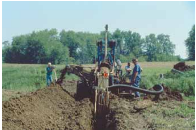
A trencher can install and remove buried field tiles. Brad Glasman
